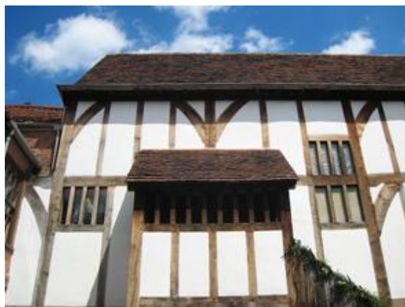
Part of the upper part of Barley Hall
